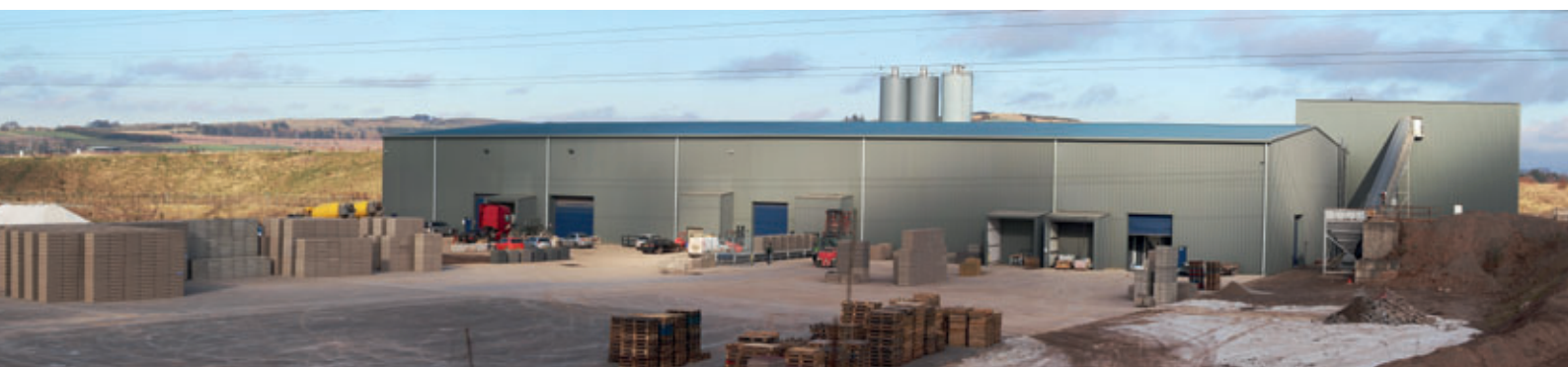
The new production hall at Laird Brothers with a 7-hectare storage yard.
