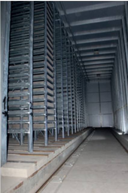
A total of 6,688 production boards can be stored at the same time in the large climatic chamber.
