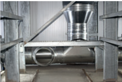
Air outlet at the bottom of the chamber. An efficient circulation system ensures a uniform flow with the precisely tempered air mixture.
