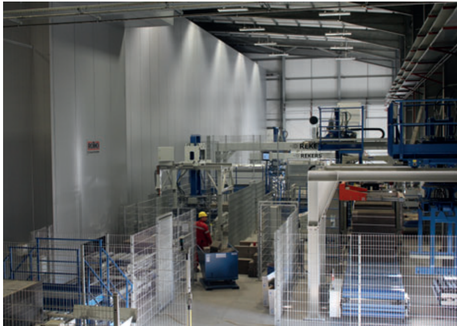
Rekers also supplied the transport and handling equipment on the dry side of the new plant.
